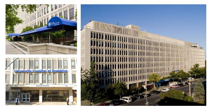
In addition to interior renovation, the recommended Current Hospital Reinvestment project includes exterior envelope upgrades. Existing windows allow excessive air and moisture into the building, which can compromise infection control and disrupt patient recovery. External envelope upgrades will address these issues and replace the existing windows with properly sealed units.
