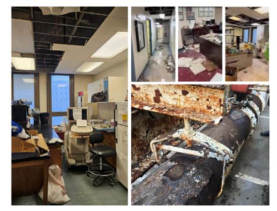
The hospital's MEP distribution systems, original to its 1966 construction, are in distress due to corrosion and/or have exceeded their expected lifespan. Several systems are at risk for failure. Comprehensive rehabilitation and replacement of MEP systems throughout the hospital will address this. 5
